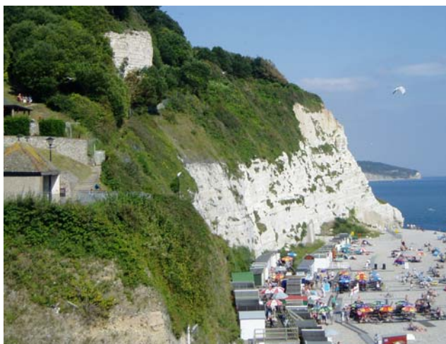
Beer Cliffs – a major and ongoing cliff works scheme
