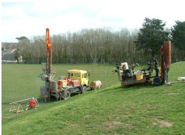
Ground investigation boreholes at Bideford College
