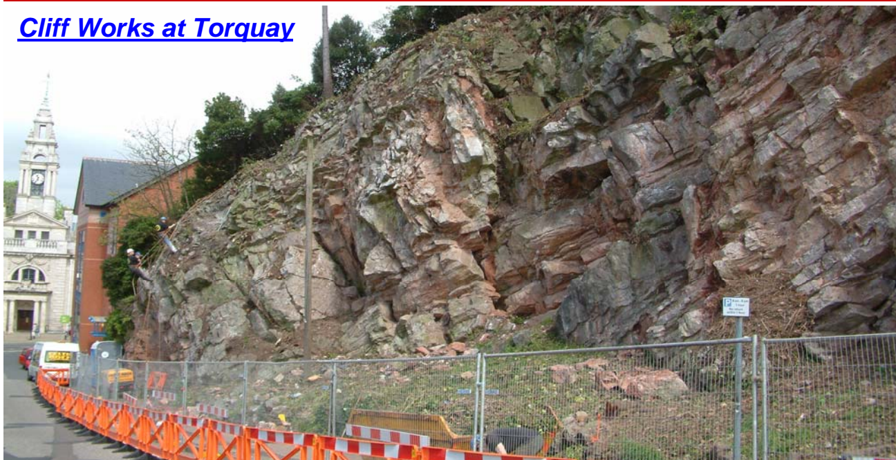
Castle Road, Torquay where the steep rock face in Devonian limestone has been investigated, trimmed and reinforced
